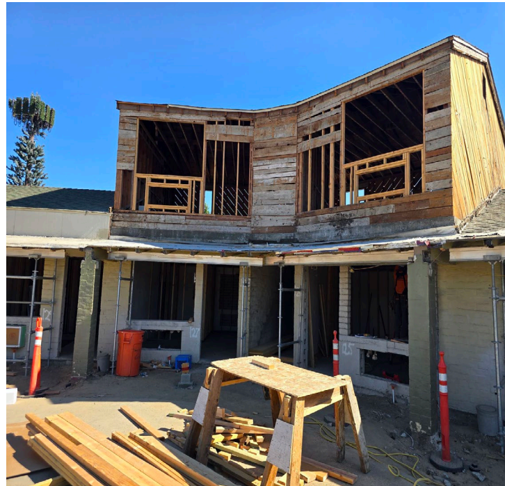
In – Progress Construction
